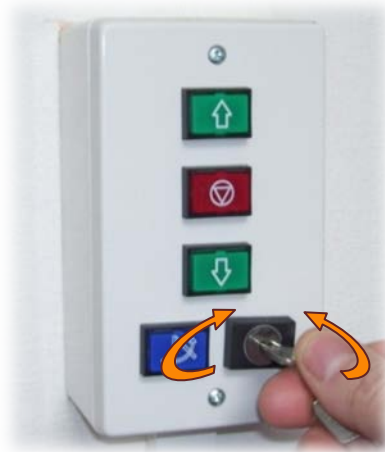
Fig 4.11.1 - Wall Mounted Hard-wired Call Station (Key-Switch and Power Door Option)
