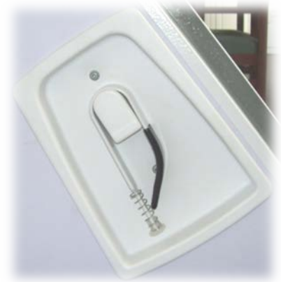
Fig 6.2 Door Release Key - (Opposite In Car Call Station)
